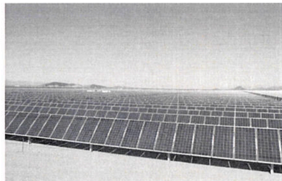
A solar array installation
