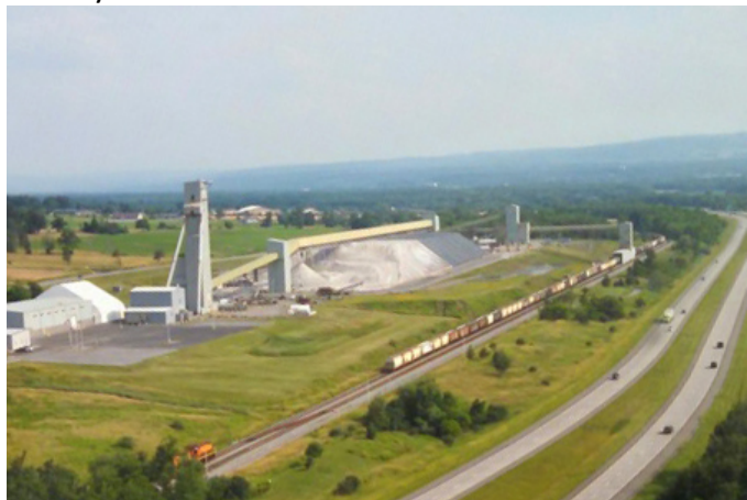
American Rock Salt facility outside of Mount Morris
