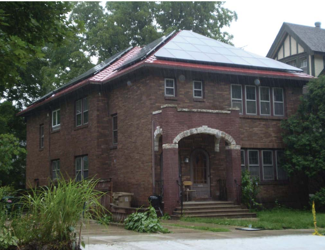
The owners of this home installed a triangular shaped PV array system so as not to compromise the design integrity of this historical home. (Vipin Gupta/PIX17930)
